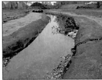
Figure 23. Log revetment / brush layering
