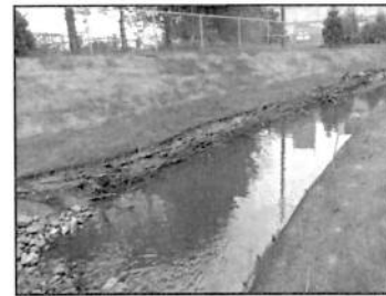
Figure 24. Brush Layering
