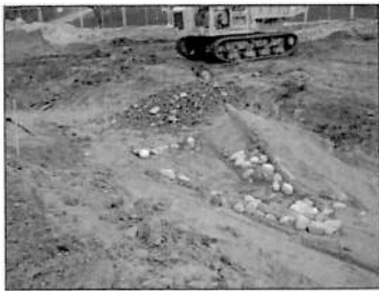
Figure 22. Log Vane
