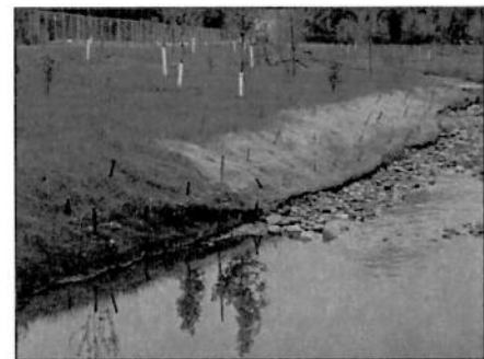
Figure 21. Live Stake Installed
